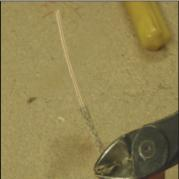
5 Cut back one of the cores so that the final crimped joints are staggered. (This will reduce the thickness of the joint.)
