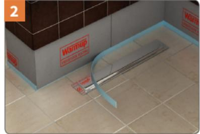
The perimeter strip should be cut flush with the tiles or levelling compound using a utility knife once complete.
