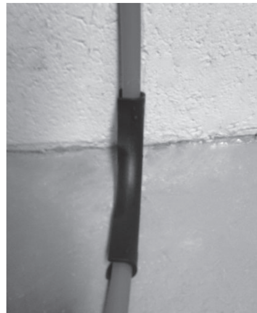
Use the Warmup Pipe Bend Support where it enters the floor.
